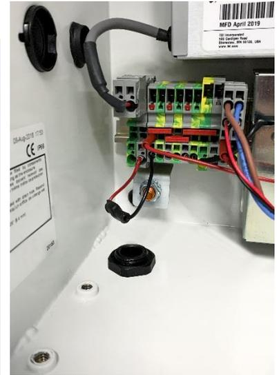
3. Insert the plastic end of GM460 probe into the sealing gland. Hand tighten the outer nut to create a seal between the gland and the plastic tubing.
